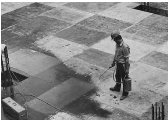
Figure 27.14 – Release Agent being applied to Soffit Form before Reinforcement is placed
