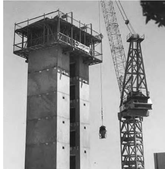
Figure 27.8 – Typical Self-climbing Formwork System
